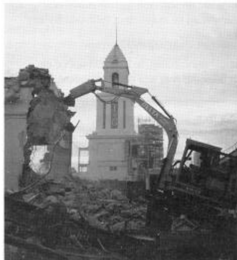
Figure 21: Machine-mounted impact hammer
