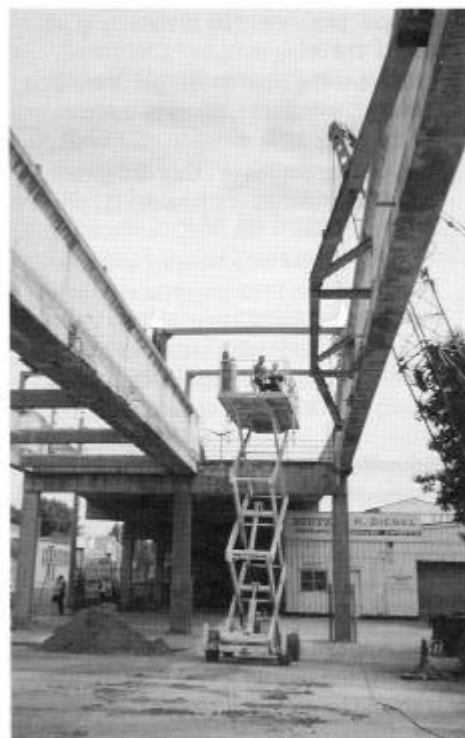
Figure 2. Scissor lift in the fully extended position.
