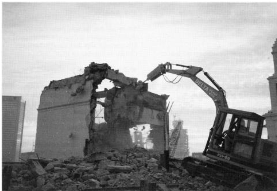
Figure 19: Mechanical Demolition
