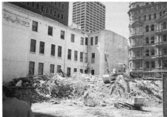
Figure 14: Removal of debris
