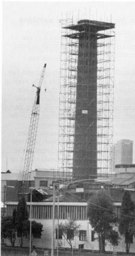
Figure 9: Heavy duty perimeter scaffolding used in the demolition of a chimney
