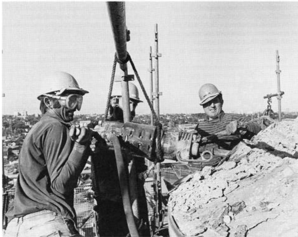
Figure 16: Pneumatic jack hammer being used to demolish a chimney. Note that the jack hammer is fitted with a silencer and its weight is supported by a rope from the scaffolding above. The scaffolding is protected by mesh brickguards to prevent debris from falling. Although the operator is wearing safety goggles and internal ear plugs the two demolition workers on the scaffold are risking serious eye and ear damage by not wearing protective equipment
