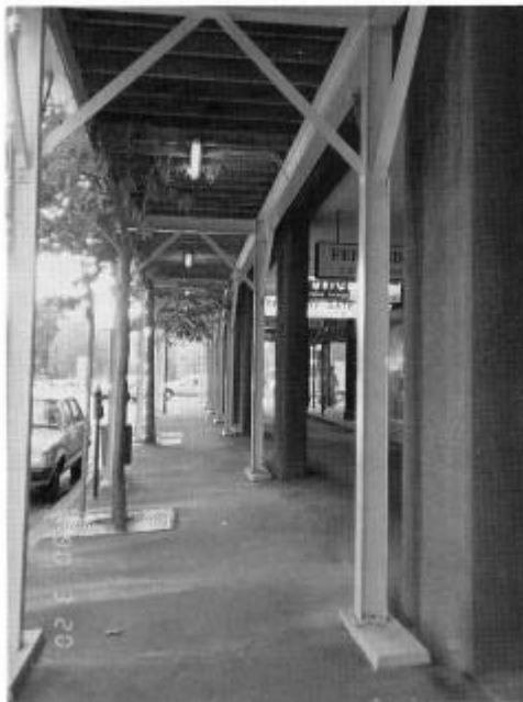
Figure 10: Scaffolding over footpath with lights
