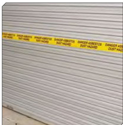
Figure 3: Barrier formed using tape (appropriate for small non-friable removal jobs or as part of system using other barriers such as hoarding).
