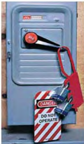
Figure 5: Locking off methods incorporating danger tags
